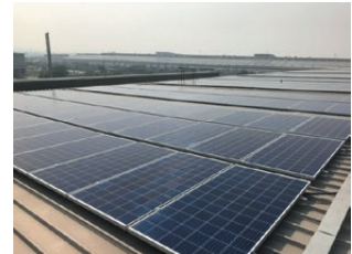
Solar power generation equipment (G-TIP)
