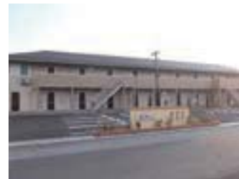
Takekawa employee dormitory (Saitama Plant)
