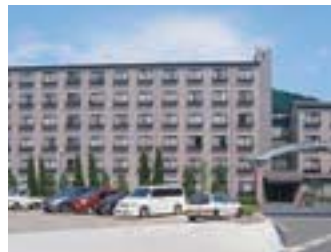
Kotoku employee dormitory (Shiga Plant)
